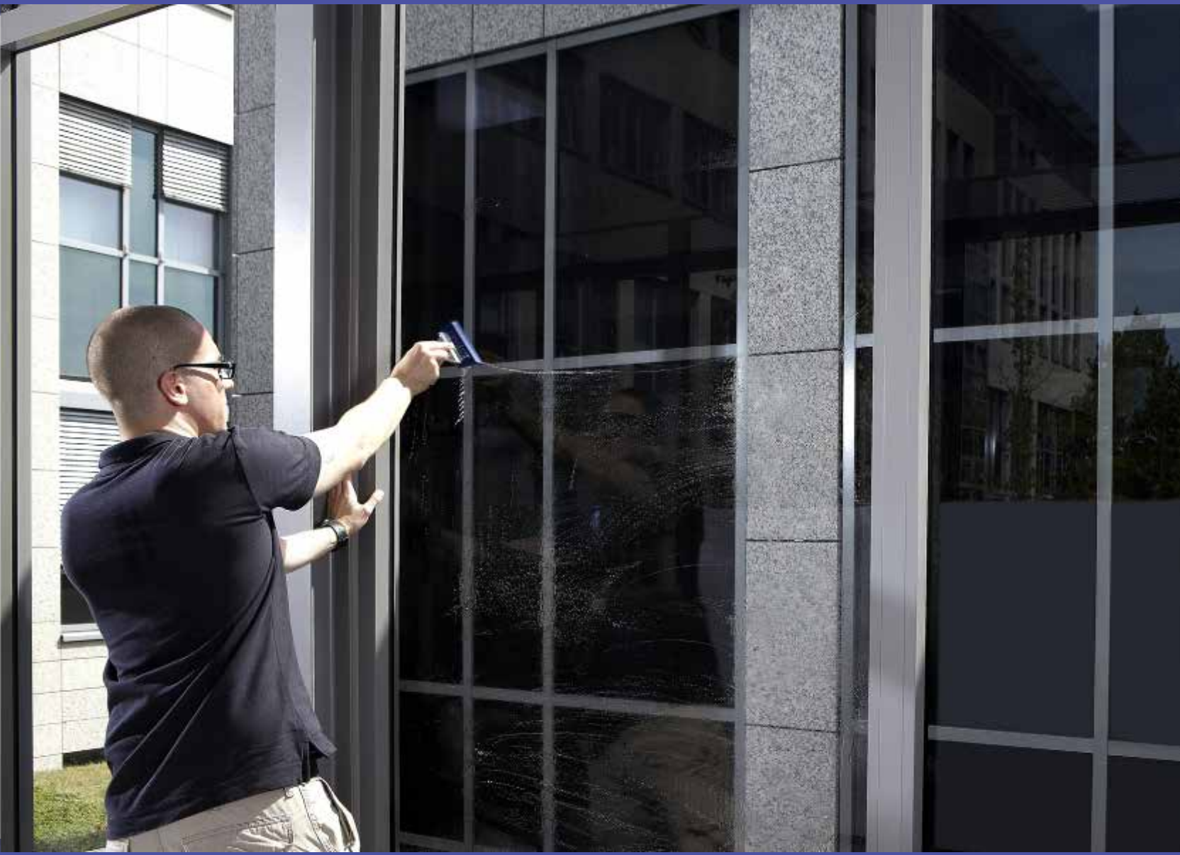
Making a perfect wet application of 3M™ Scotchcal™ Clear View Graphic Film 8150 | Step 4:
