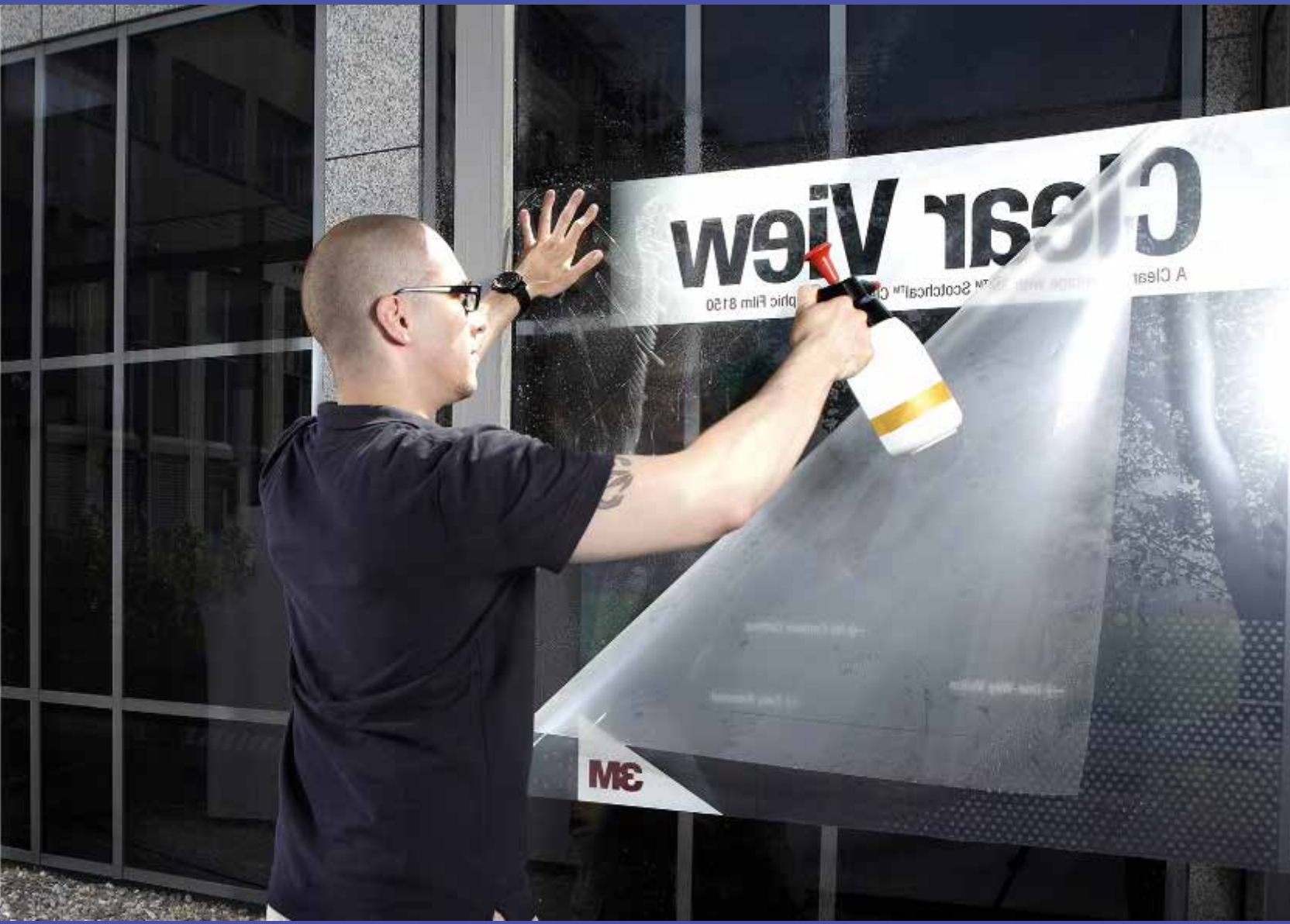
Making a perfect wet application of 3M™ Scotchcal™ Clear View Graphic Film 8150 | Step 8:
